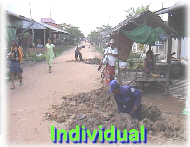
Install Main Pipes
